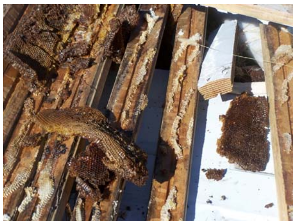
Inside the exposed column
