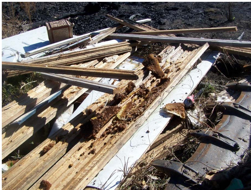
Bulldozer blade at edge of damaged column
